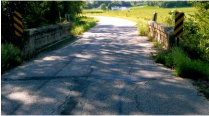
Skinner Road Bridge built in 1924
