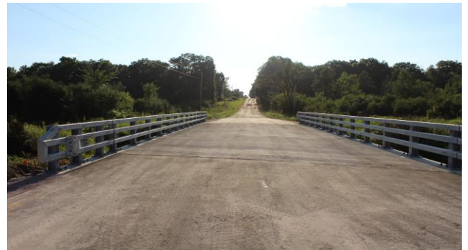
Bass Road Bridge replaced 2025
