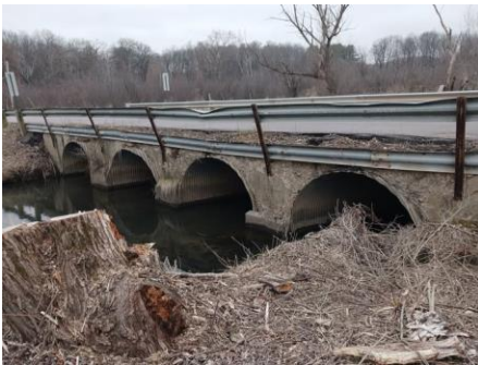
Bass Road Bridge built in 1930
